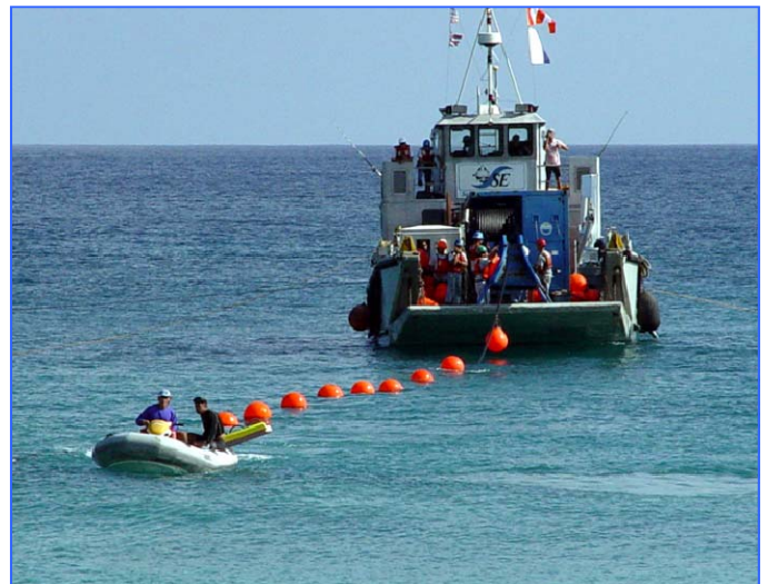
Undersea Cable Deployment in Hawaii
