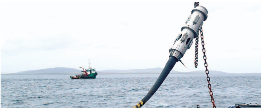
▲ Offshore Orkney: The MacArtney Inline Termination is taken onboard for assembly. The entire process takes less than two hours
